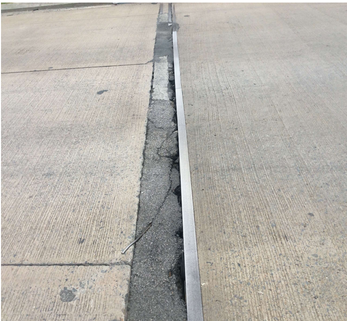
PHOTO 1 Description Bent 5 spalls filled with asphalt in the top of backwall
